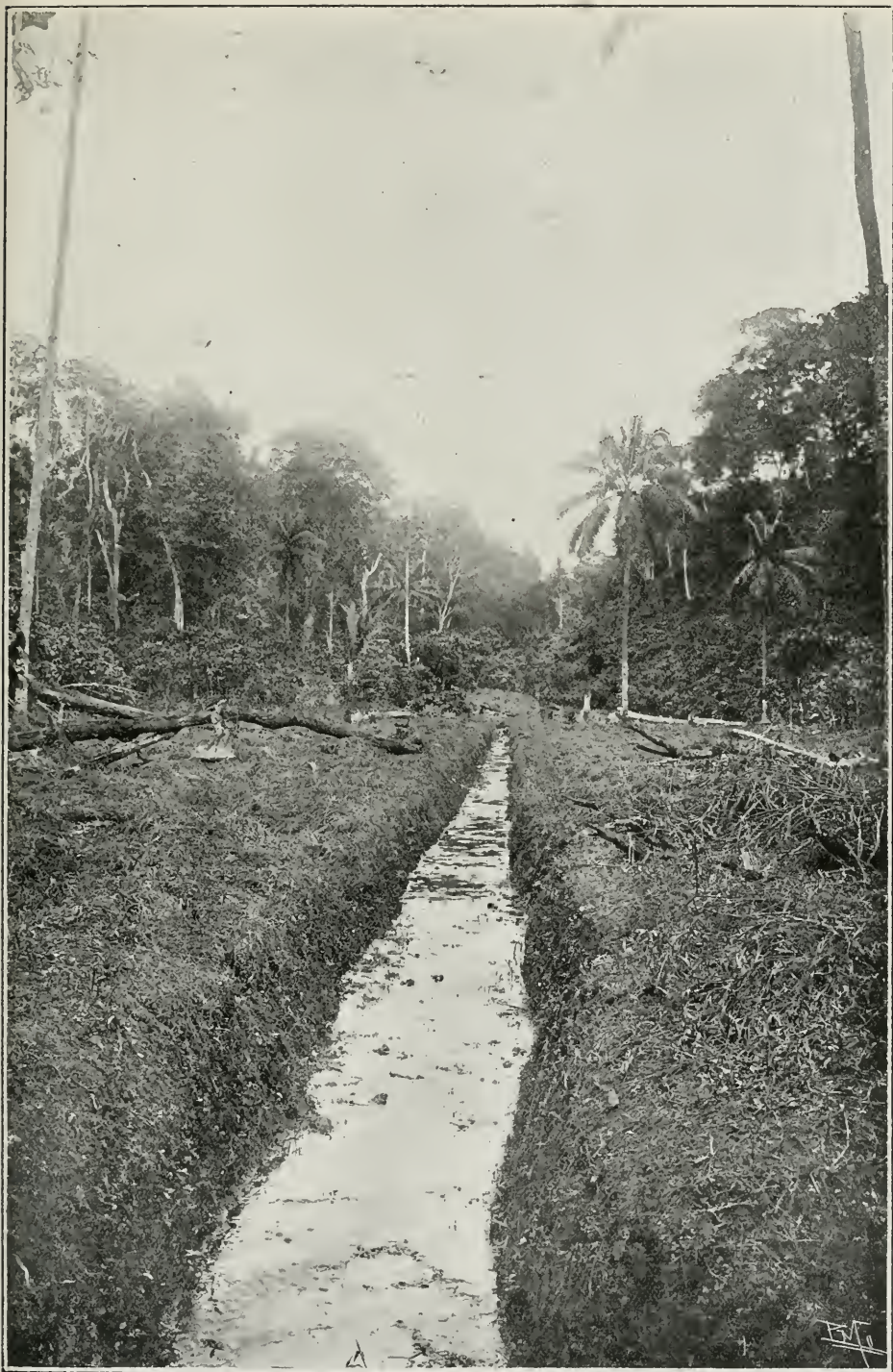
FIG. 37.—DRAINAGE WORK: ON SWAMP OF BOA-VISTA, ROÇA SANTA RITA.
